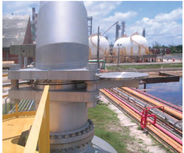
Cam-Set DN 500 (20"), ASME 150# with spectacle plate support
